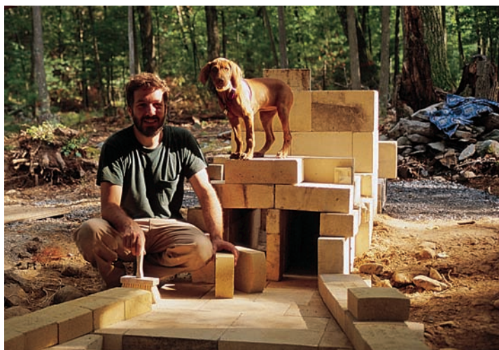
Constructing the anagama: once the floor and flue opening were complete, Rowan began setting the arch.
