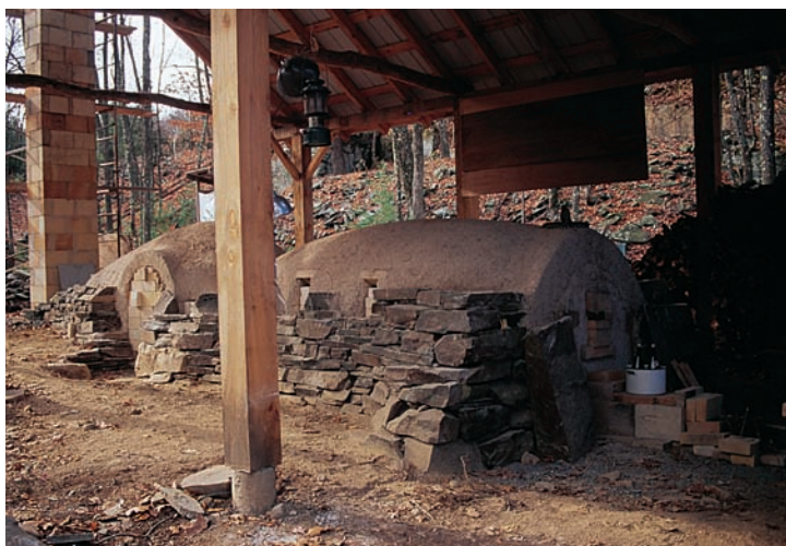
Buttressed with local stones for insulation, the new kiln is ready for loading and firing.
