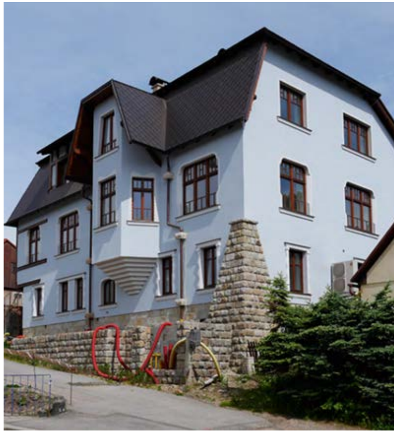
Sladkovského 545: The Kohn house in various stages of recent restoration work, seen by me in 2014 and by Noah and Julia in 2016.
