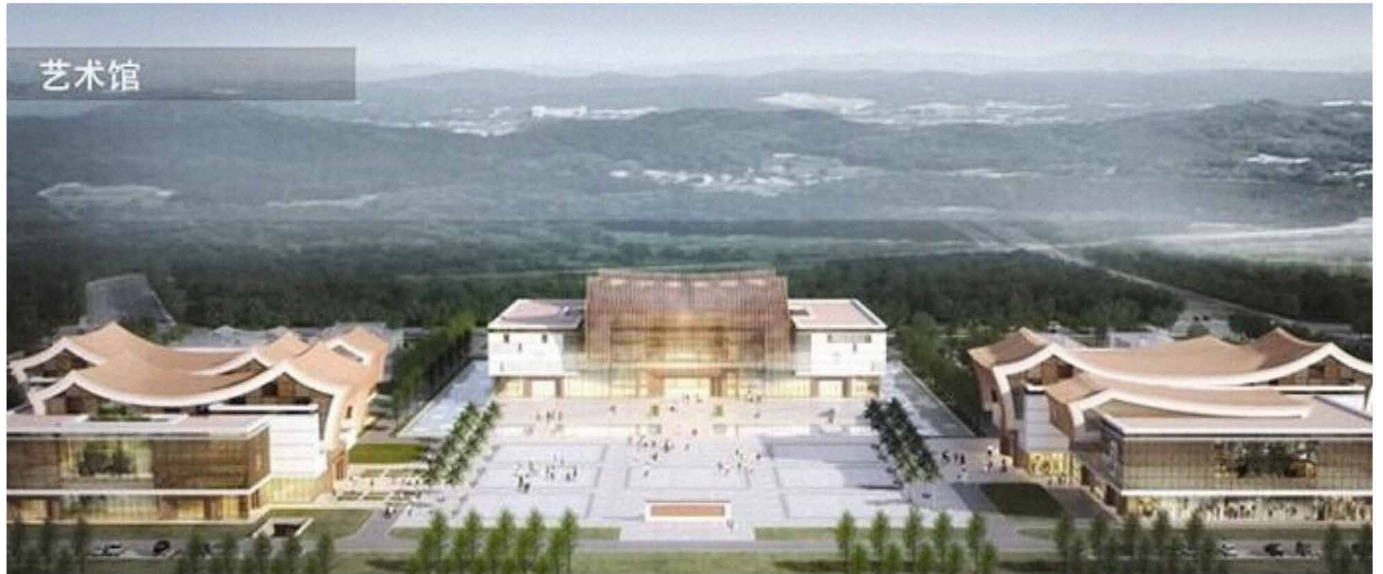
Zhangzhou Museum of Art under construction
